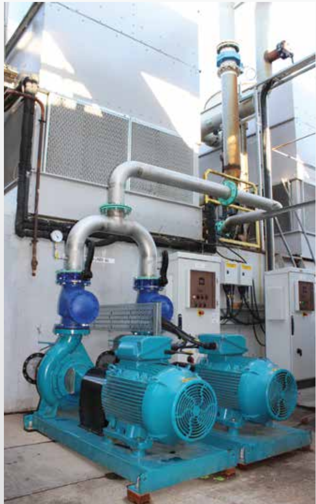
Installation involved core drilling the tower bunds and inserting valves and pipework, followed by installation of the Aturia pumps and variable speed drives.
